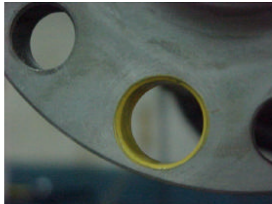
FIGURE 14 CORE SAMPLE HOLE AFTER APPLICATION OF ZINC CHROMATE PRIMER
